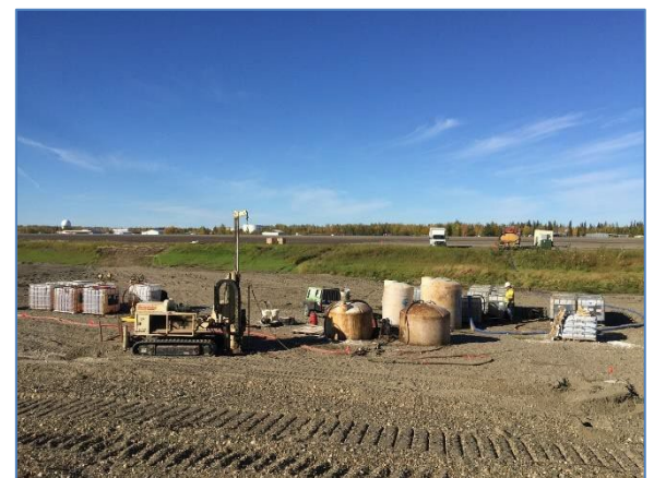
Groundwater remedy at Site SS015 using emulsified vegetable oil injection to biodegrade chlorinated solvents.
