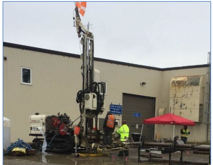
Installing monitoring well for PFAS investigation using sonic drill rig.
